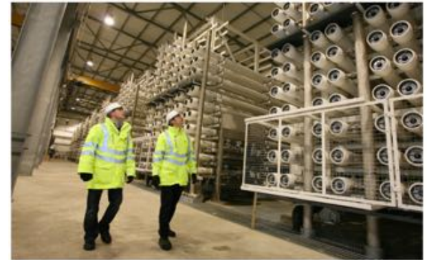
The Beckton desalination plant provides water for 400,000 households by reverse osmosis membrane filtration
