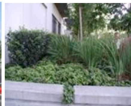
Building Bioretention Planters (Portland, Oregon, USA)
